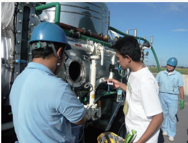
Practical explanation and inspection of Johkasou system
