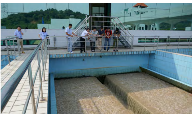
南京市城北浄水場砂ろ過池現場 (逆洗時の風景) The site of Nanjing Chengbei Water Purification Plant (scene of sand filter backwashing)
