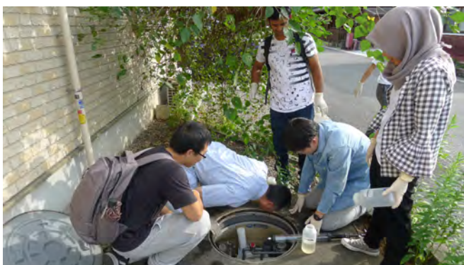
Field study on Johkasou 浄化槽の現場研修
