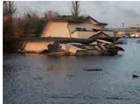
Damage to Buildings (above) and Damage by Floods (below), as Results Affected by Land Subsidence
