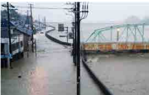
Flooding of the Kumano River (Kiho Town, Minamimuro District, Mie Prefecture) caused by Typhoon No. 12 in 2011c
