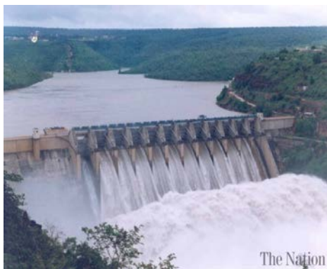
Construction of reservoirs
