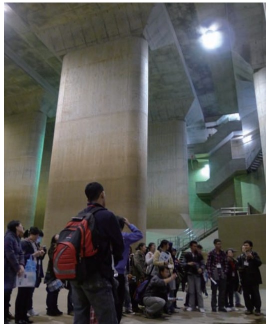
In the water discharge tunnel on the outskirts of the Tokyo Metropolitan Area
